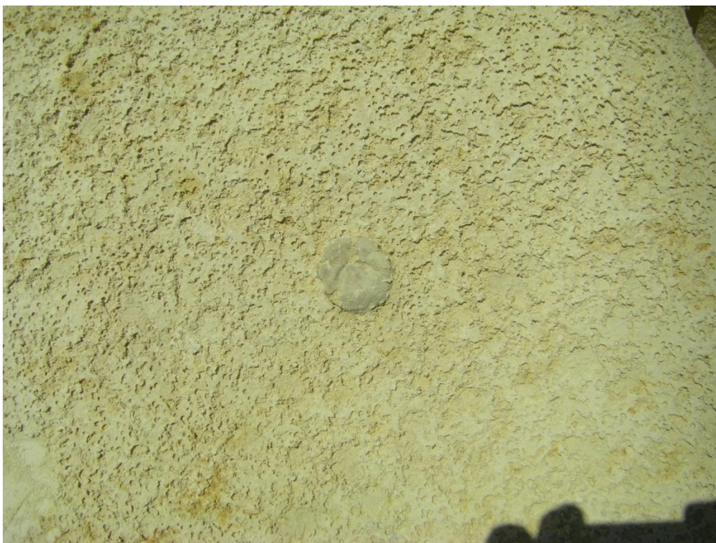
Figure 11: Photograph showing typical weathering of Upper Globigerina Limestone at il-Kalanka T0Tawwalija by flaking
